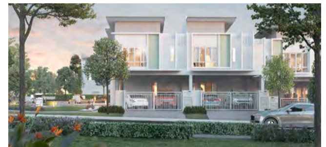
The units have a chic, modern facade that embodies harmony with their environment.
