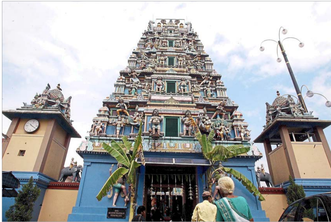
The central tower aims to reconstruct the appearance of the gods' mountaintop dwelling.
