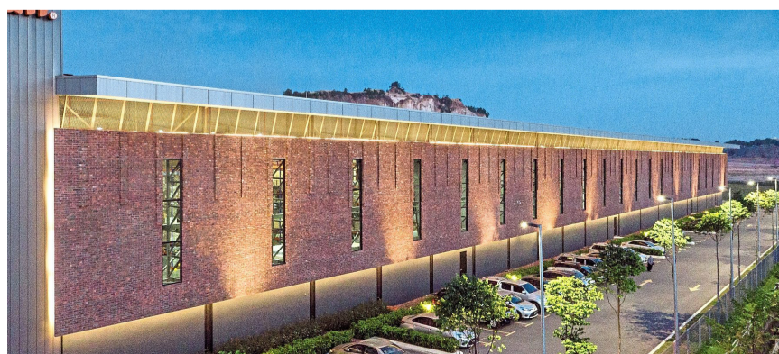
The suspended brick wall serves as both a wind funnel and heat trap for the warehouse, and has narrow and thin windows to reduce heat penetration.
