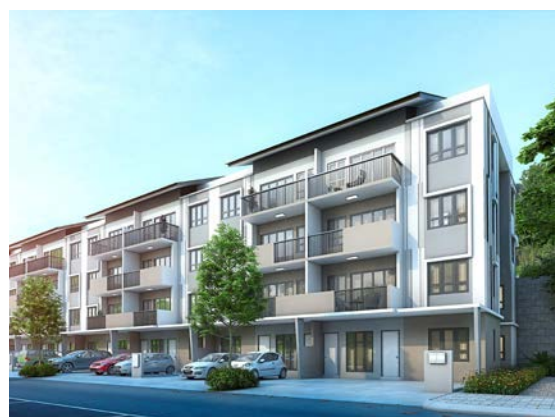
The front view of the four-storey townhouses.
