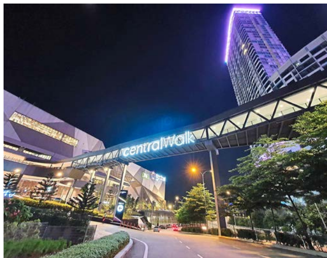
Excellent connectivity with pedestrian linkage to offices and shopping amenities. LRT3 i-City station is just minutes walk away.
