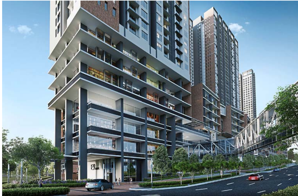
The covered link bridge from Emerald 9 shelters residents from heat and rain while linking them directly to the MRT station.
