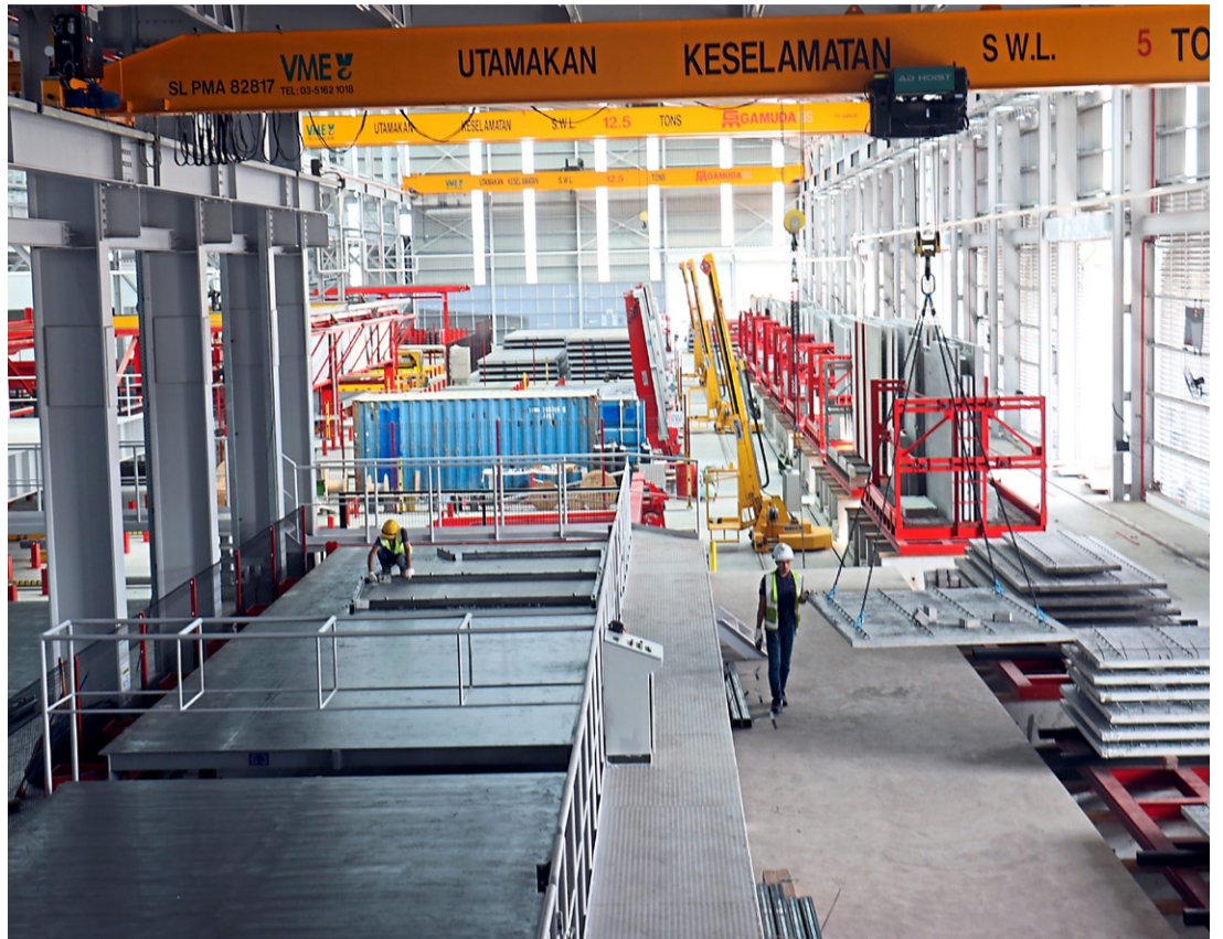
IBS manufacturing plants, such as Gamuda's facility in Banting, combine the planning efficiencies of BIM with the cost savings of prefabrication to drastically lower the cost and delivery time of buildings.
