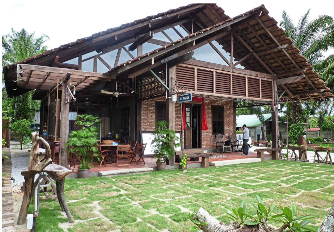
Reclaimed wood and other building materials can be re-used imaginatively in contemporary homes. Note the double roofs that aid thermal dissipation and the gable windows that maximise natural light to reduce electricity consumption for cooling and lighting.
