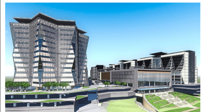
3D visual of the Parcel F project generated by Sunway Construction Virtual Design and Construction (VDC) or most commonly known as Building Information Modelling (BIM)
