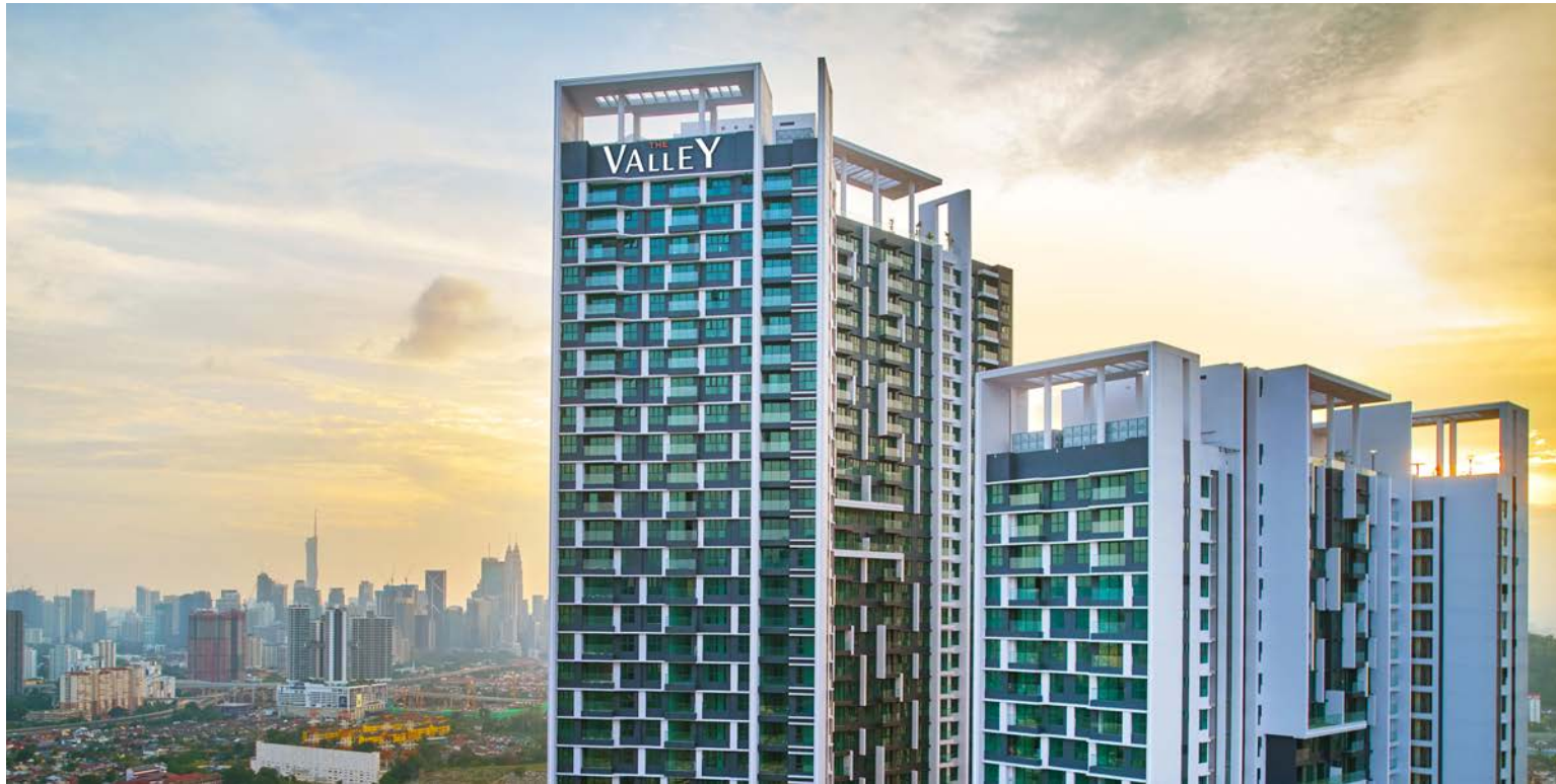
SkySierra Residences (The Valley) stands as SkyWorld's tallest building to date, also achieving the company's highest QCLASSIC score at an impressive 86%.
