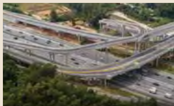
FEDERAL HIGHWAY DIRECT LINK
