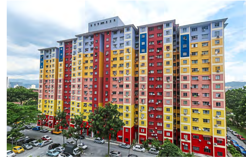
Apartments can reduce electricity consumption by facing the parts with the biggest surface area in a North-South direction.
