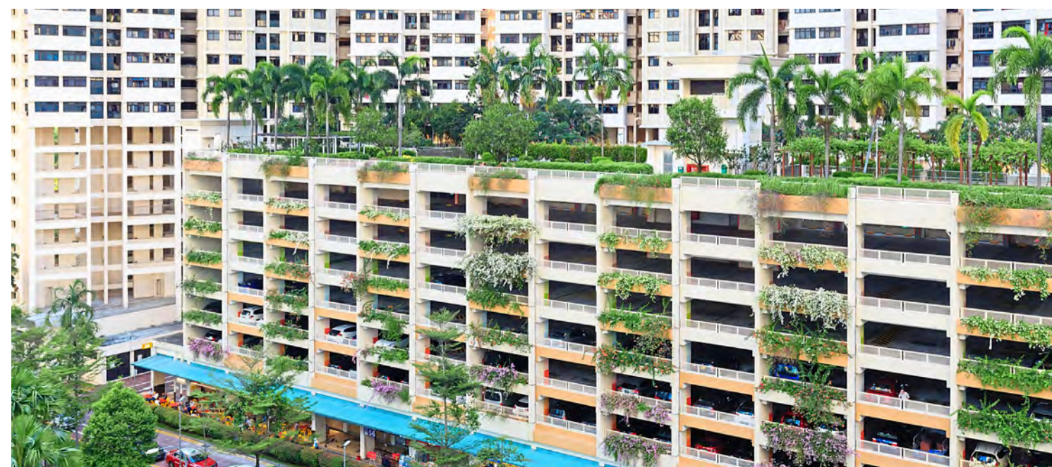
The usage of plants on the balconies and rooftops will help reduce heat build-up.
