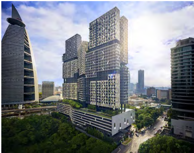
Eupe's first project in Kuala Lumpur is Novum @ South Bangsar, which was completed in 2020.
