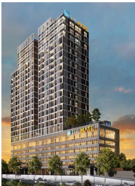
The Mate utilized Building Information Modelling (BIM) technology in its construction process.
