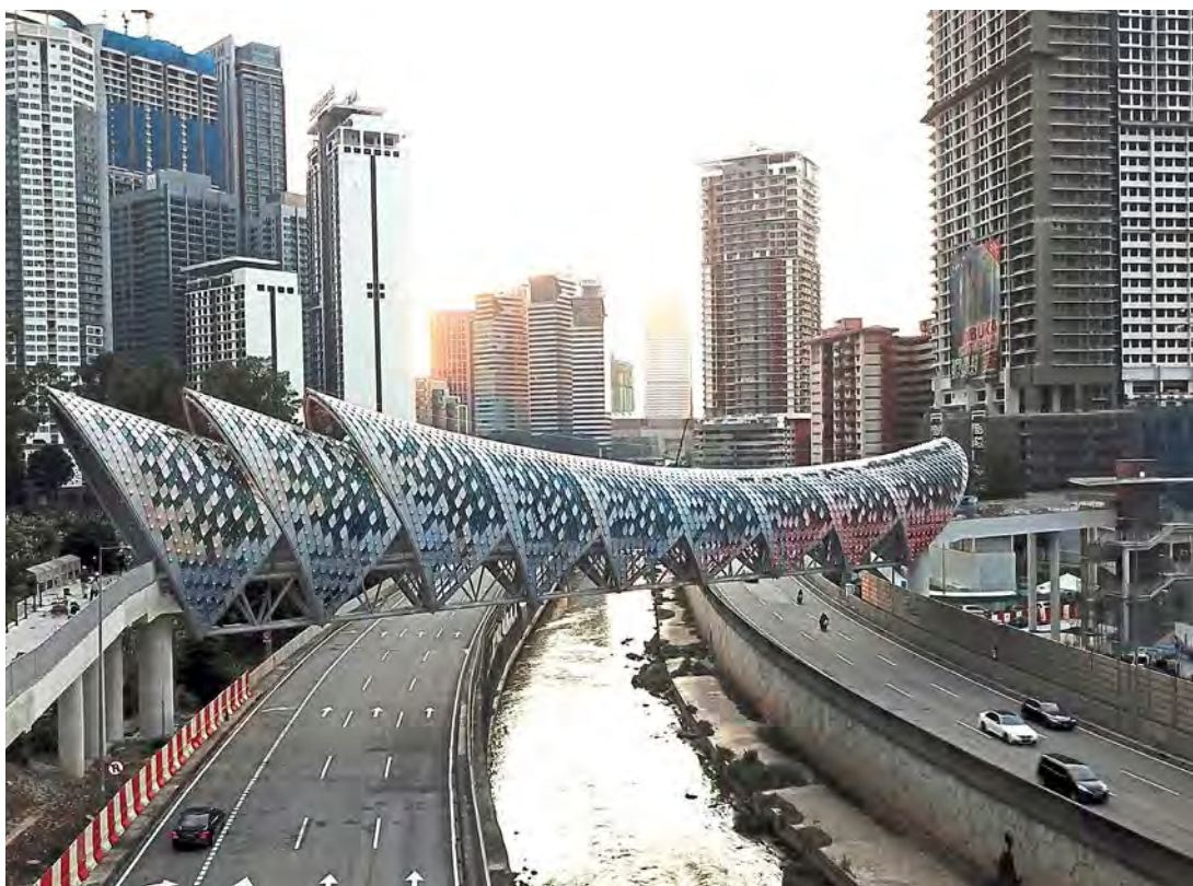
BELOW The Saloma Link allows that marriage between the old and new parts of KL, with Jalan Ampang on the left, and Kampung Baru on the right. The 69m pedestrian bridge crosses Akleh and Klang River to open up so many exciting possibilities.
