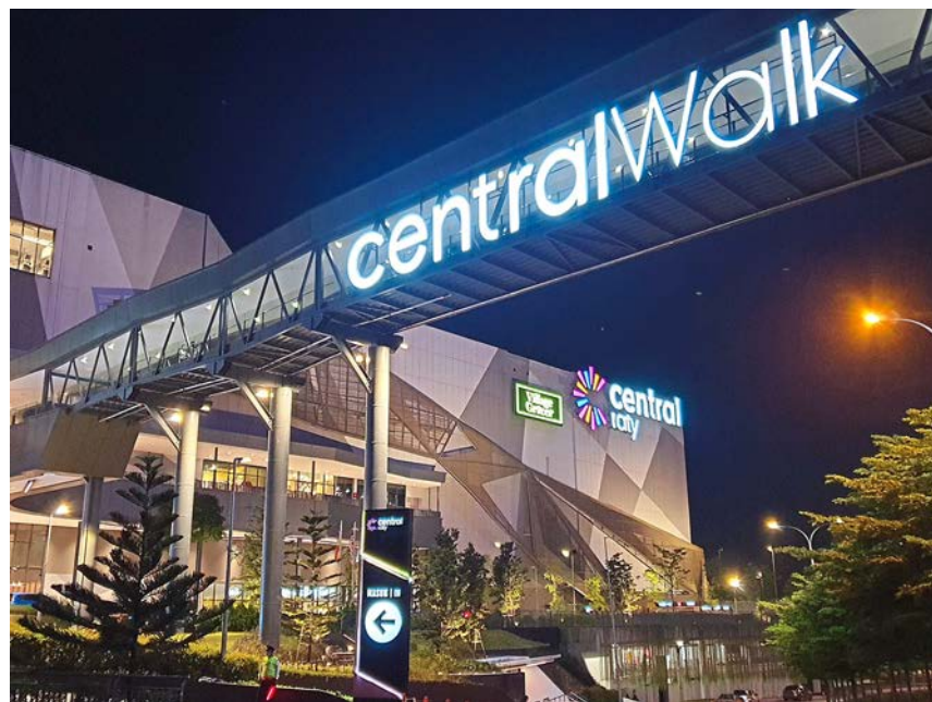
The elevated interconnecting bridges and linked walkways in i-City SGT provide easy and safe access to the residences, offices, hotel and shopping venues.
