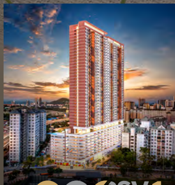
PSV1 RESIDENCES PLATINUM SOUTH VALLEY
