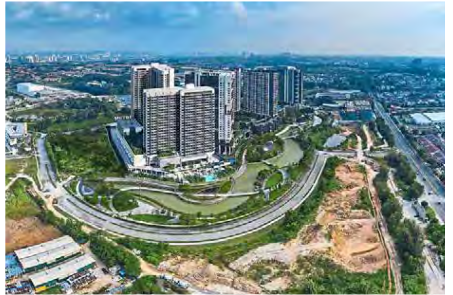
Aerial view of the 9.2-acre central park from Alira @ Metropark Subang.
