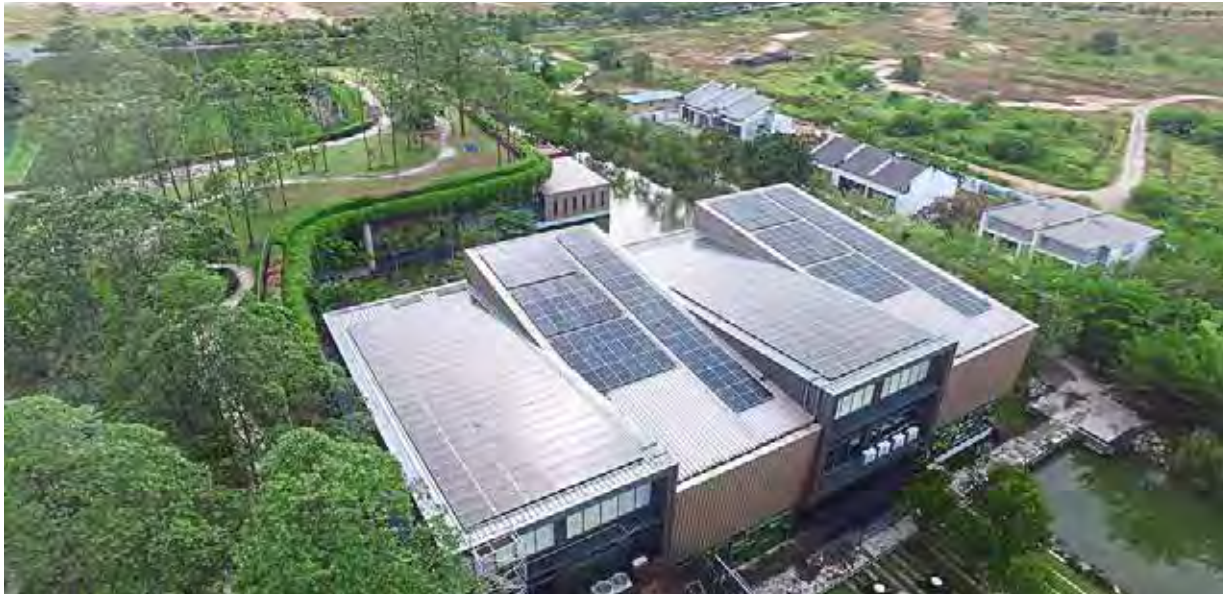
Solar panels installed at The ARC, Bandar Rimbayu, Selangor.
