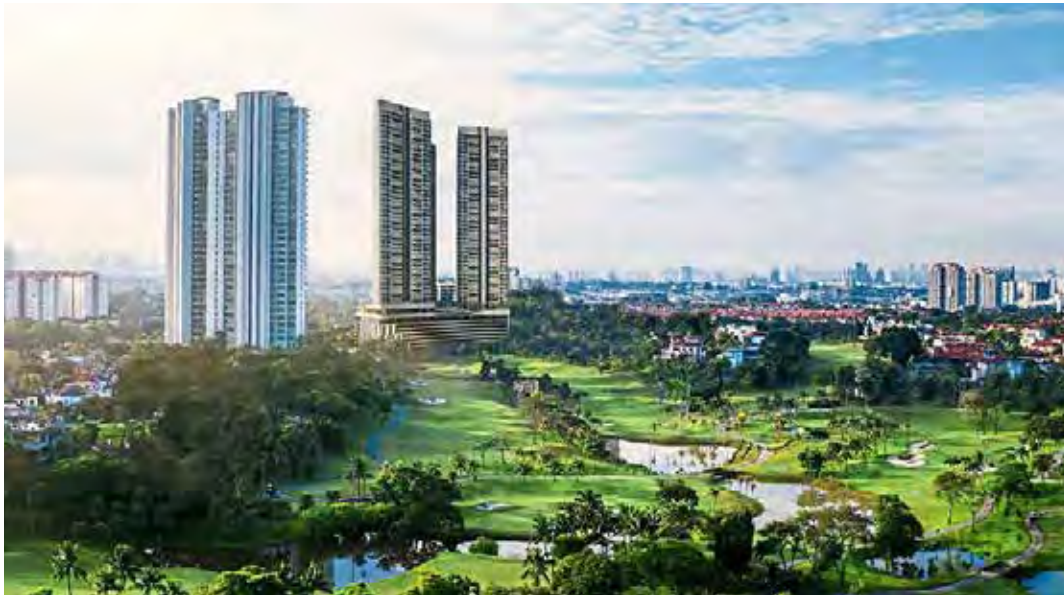
Panoramic view overlooking the golf course from Aetas Damansara.
